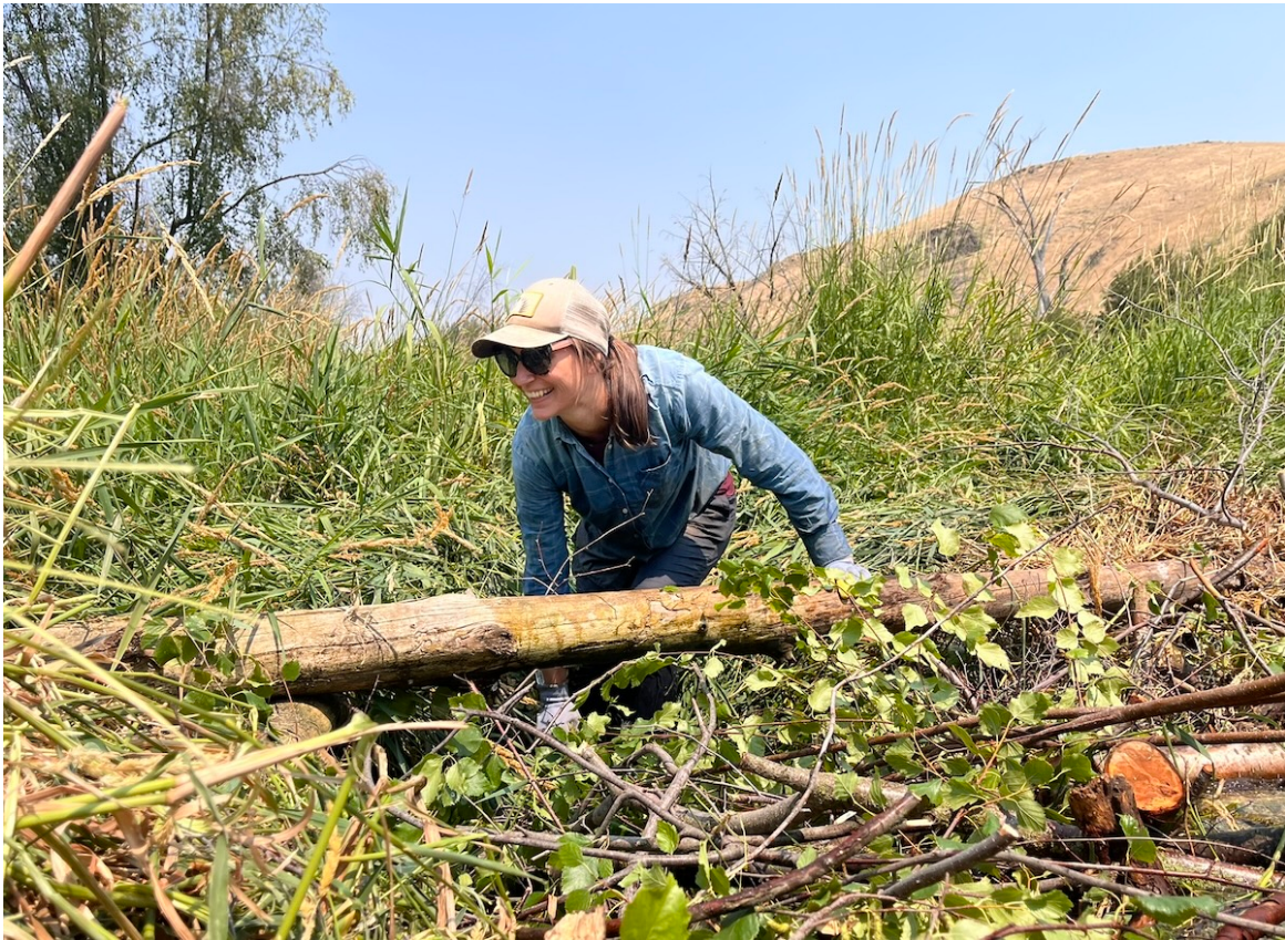
A smiling volunteer places a log during the construction of a post-less beaver dam analog on the Wallowa River.
