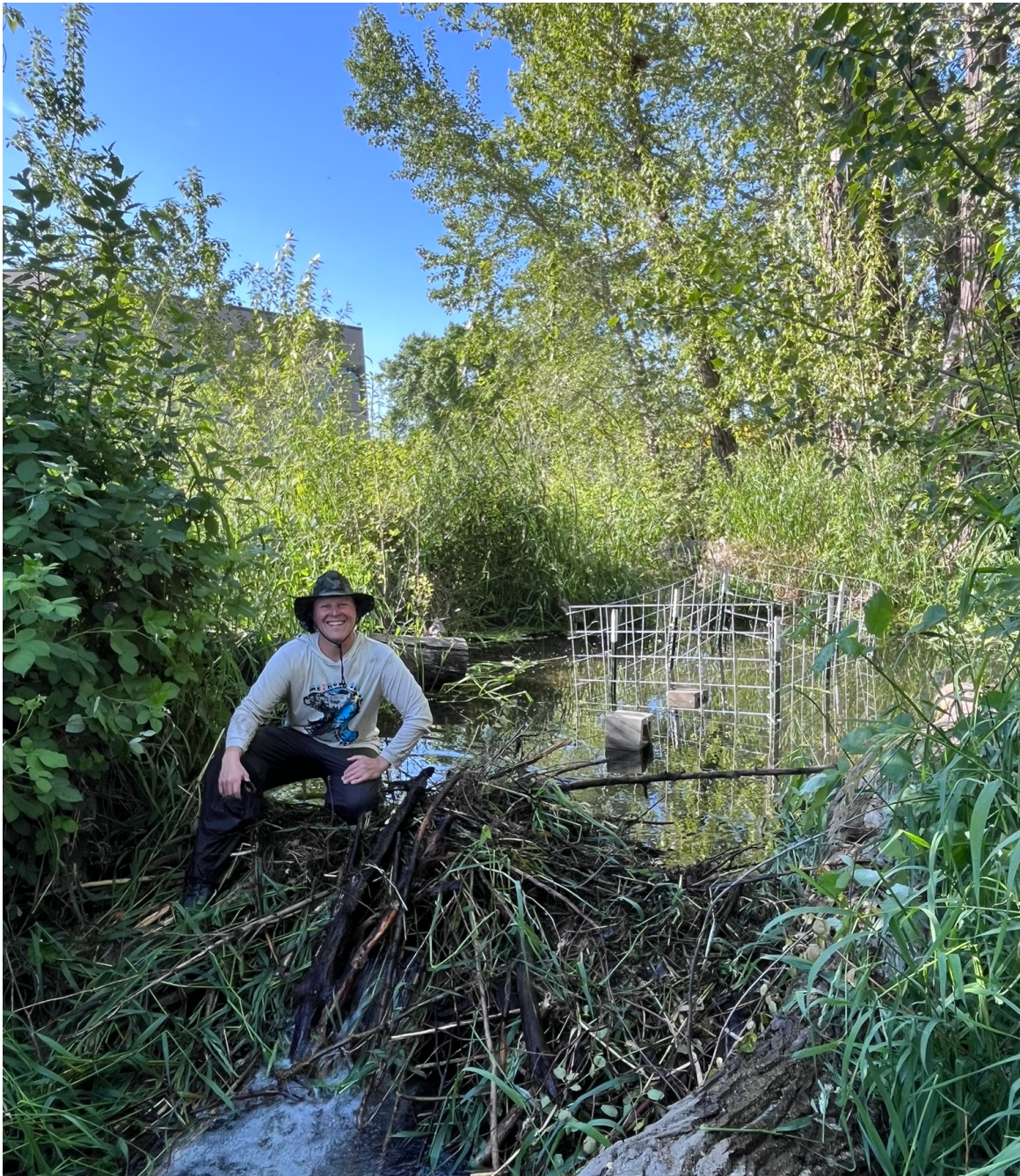
Stewardship Manager Ian Wilson on-site at Walla Walla Community College, pictured here next to the pond leveler installed by the team.
